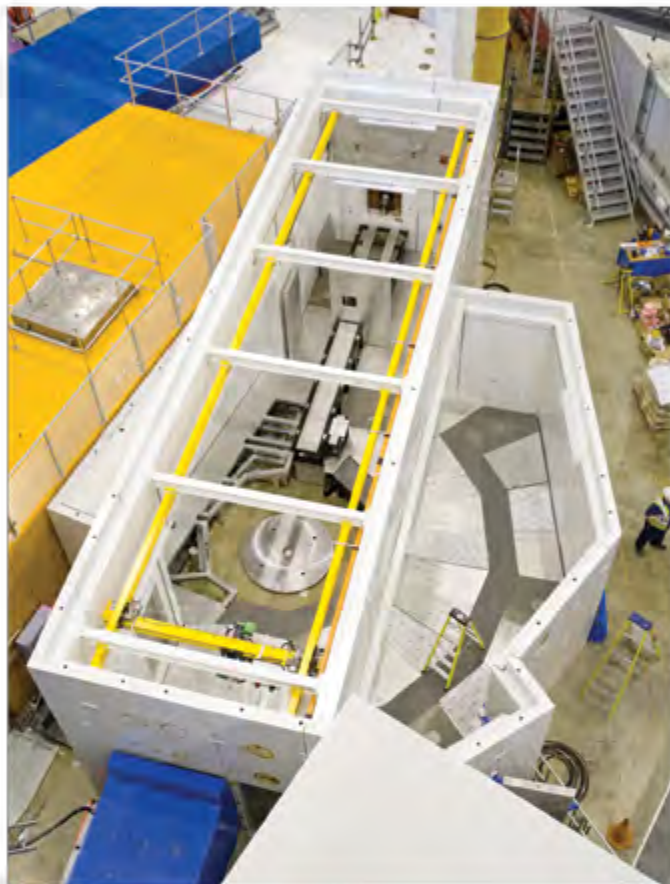
Above: The inside of the Larmor blockhouse. The raised floor contains a granite section that will be used to allow the large detector bench to rotate around the sample position from 0 to 135 degrees on an air-pad system.
