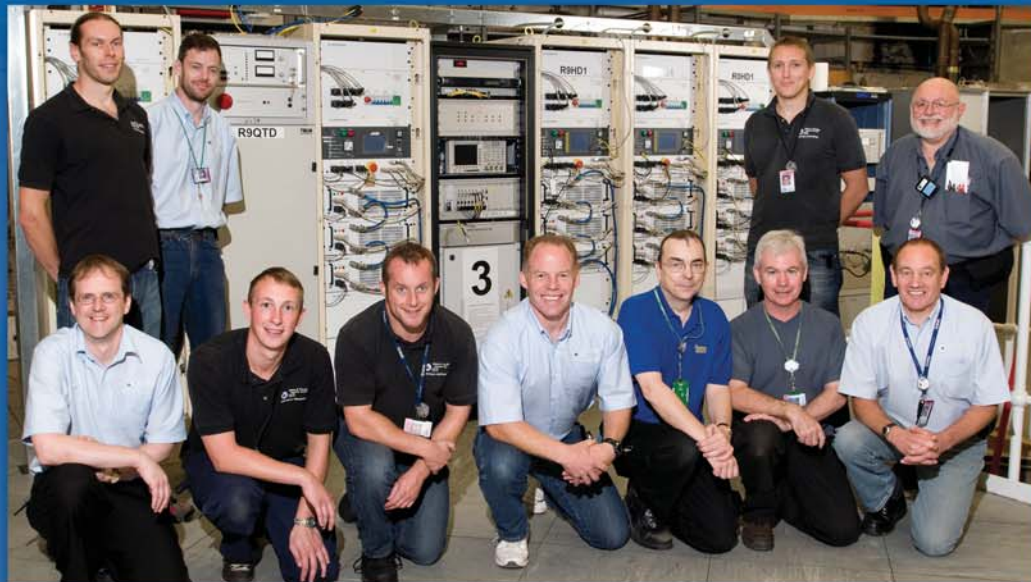
Team involved in the installation of the 180kW Bipolar pulsed power supplies for the synchrotron trim quadrupole and steering dipole magnets.
