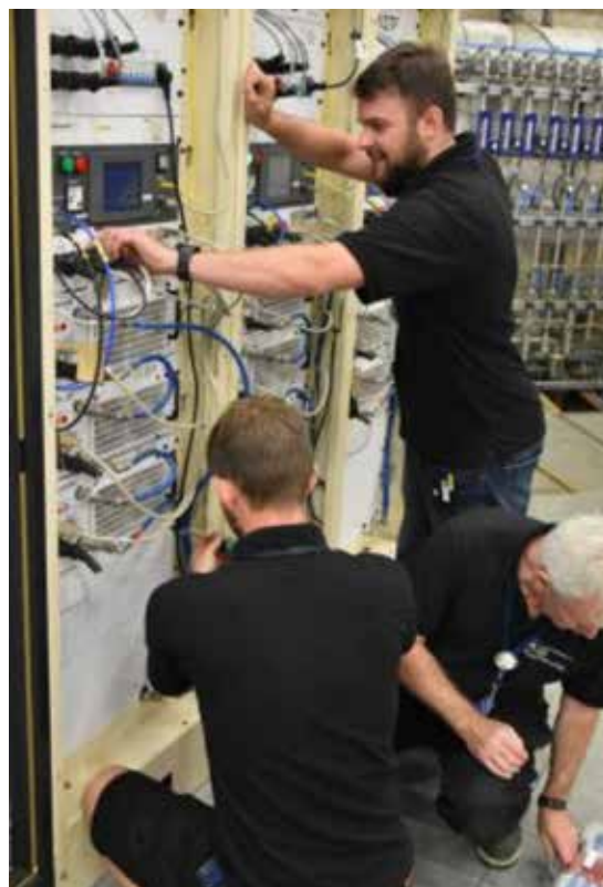
Magnet power supplies group staff Jaysen Tydeman, Michael Julian and Noel McNamee, installing a trim quad filter unit.
