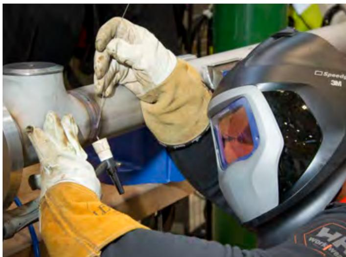
Phillip Lester about to perform a TIG weld on pipework.
