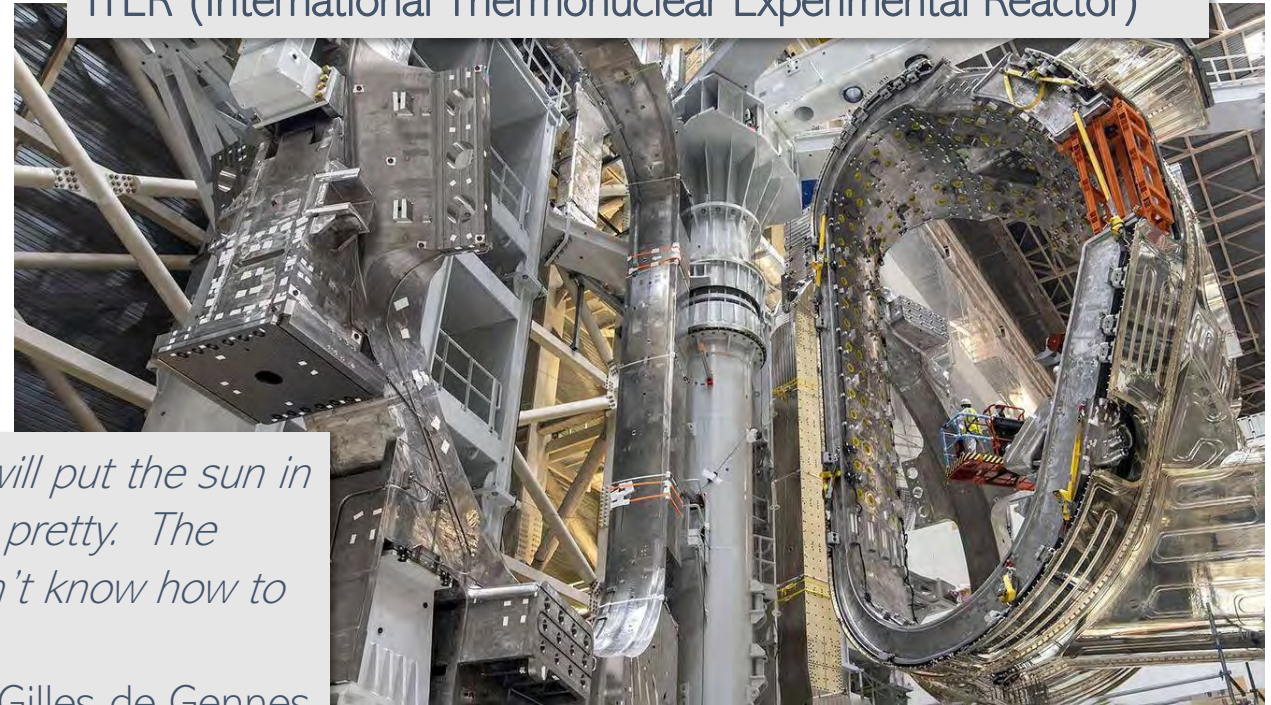
ITER (International Thermonuclear Experimental Reactor)
