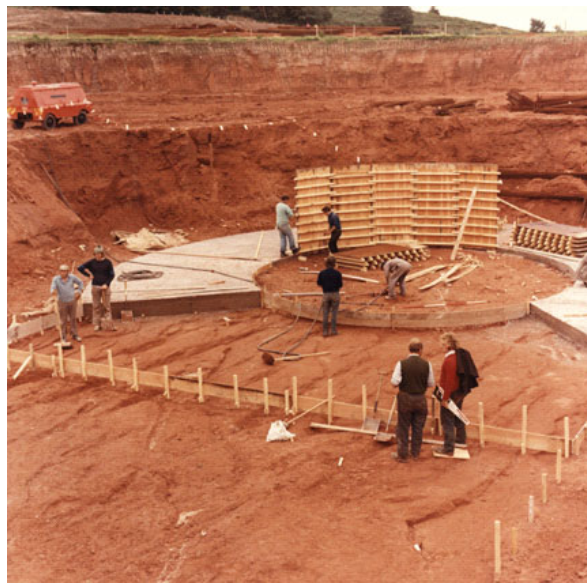
Figure 14.5 The concrete foundations for the Nuclear Structure Facility being cast directly on to the Bunter sandstone on the Daresbury site
